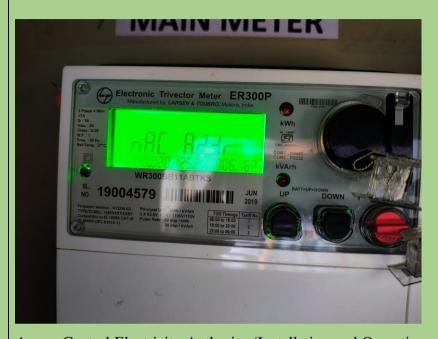
As per Central Electricity Authority (Installation and Operation of Meters) (Amendment) Regulations, 2019 clause 14 (i)-b "All Interface Meters shall be tested on-site using accredited test laboratory for routine accuracy testing at least once in five years and recalibrated if required.
